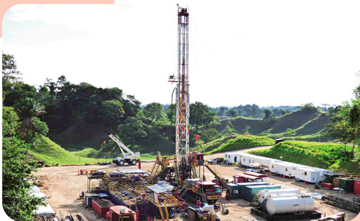
Foto: Service King 775, Torre 6
